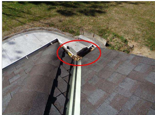
1.5 RAIN GUTTERS / EAVESTROUGHS Picture 5
