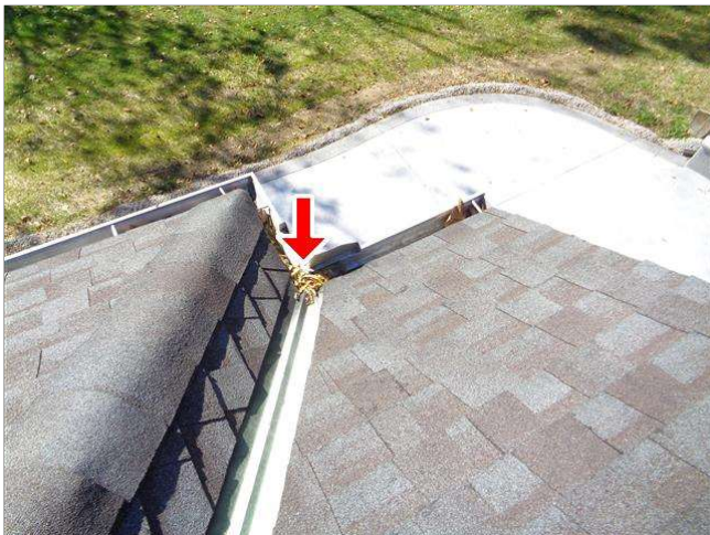
1.5 RAIN GUTTERS / EAVESTROUGHS Picture 4
