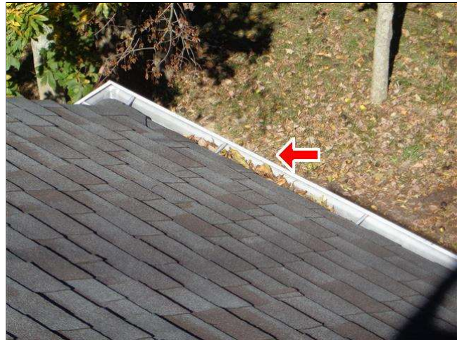
1.5 RAIN GUTTERS / EAVESTROUGHS Picture 3
