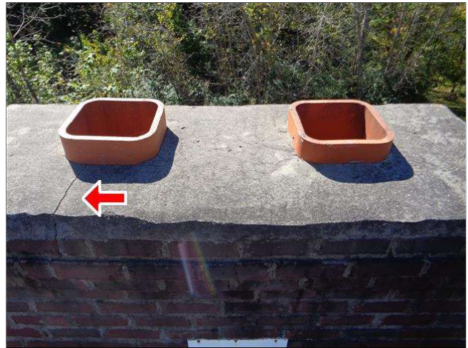
1.1 CHIMNEYS / VENTS #1 Picture 1
