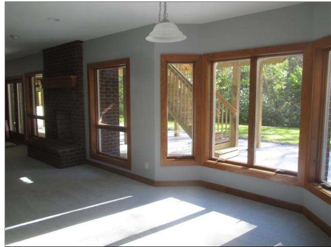
9.0 FOUNDATION WALLS Picture 4
