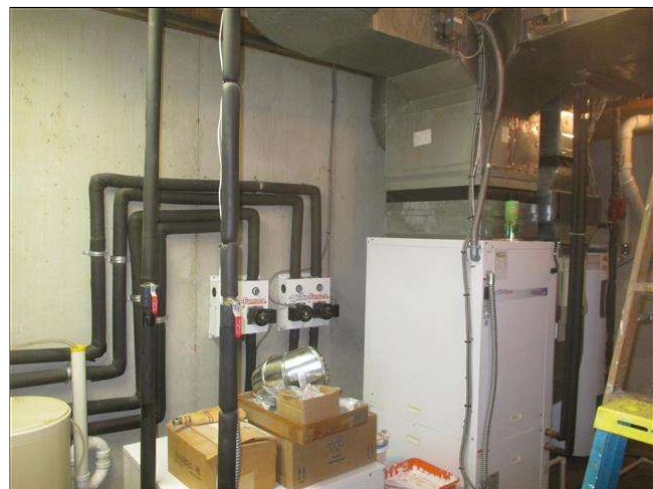
9.0 FOUNDATION WALLS Picture 6
