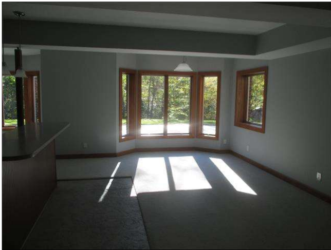
9.0 FOUNDATION WALLS Picture 3
